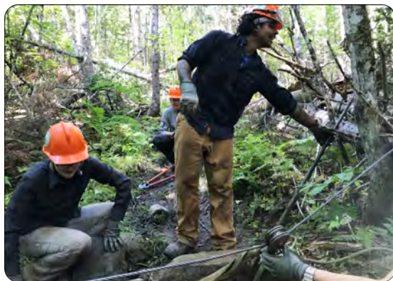
Using the Grip Hoist at Marble Brook
